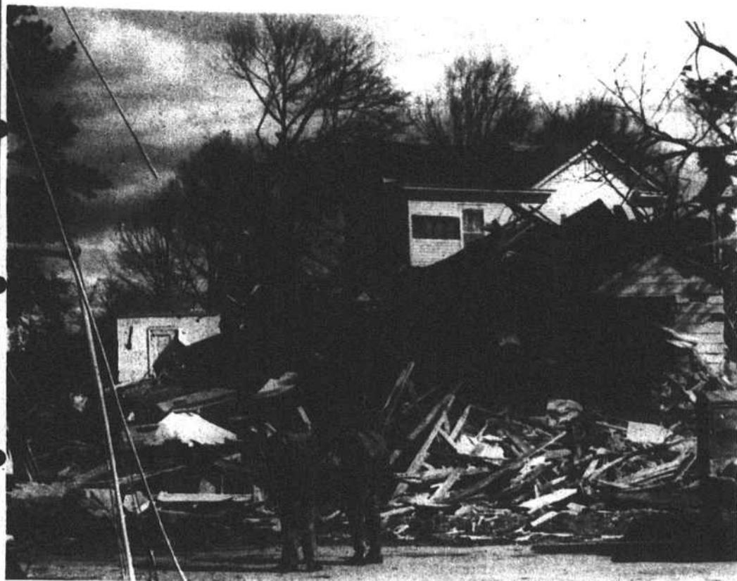
Examining the wreckage
