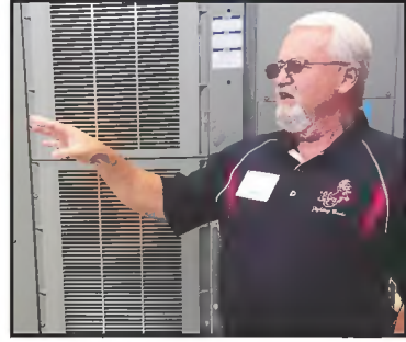
Facilities director Charles Tapp with a chiller.
