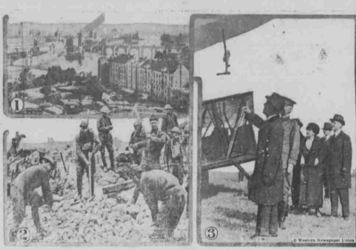
1—General view of Prague, capital of the new Czech-Slovak republic. 2—American engineers and infantrymen establishing a road in preparation of Prague. 3—President Wilson inspecting an American Handley Page biplane which flew from Miler's to Washington, 230 miles, in three hours.
