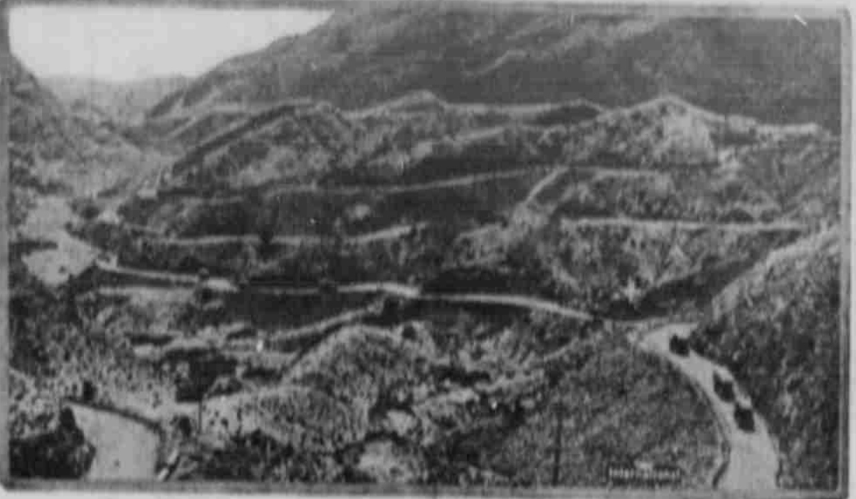
View of the roads ascending the Khyber pass, looking toward the plateau of India. The upper road is the old camel caravan road leading into Afghanistan. The lower road was specially constructed last year by British engineers for motor transport.
