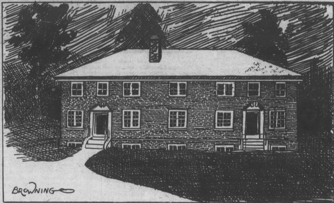
The above drawing, sketched from an actual photograph, shows the newly completed nurses' home at Hugh Chatham Memorial hospital. Constructed at a cost of over $20,000, the new building is modern in every way. It is located a short distance southeast of the main hospital building.
