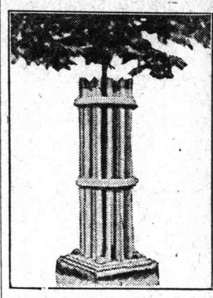
age or house coloring. When the tree outgrows its narrow box, it is no great matter to remove the concrete and release the steel bars. While the first cost is somewhat higher than a good wooden box, the lasting qualities of the concrete make it worth while.-Popular Mechanics.
