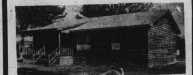
N. Frisco St.-3 bdrm., 2 baths, outside storage, spacious lot w/garden spot, reasonably priced.
