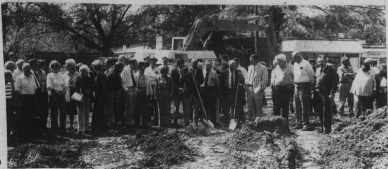
ROUNDBREAKING - Approximately 200 people gathered at the corner of Central Avenue and Walnut Street in Pink Hill for the official groundbreaking of the new Pink Hill Medical Center. Construction of the 2,700 square foot facility began recently by Farrior & Son of Greenville. The building includes a reception area, two business offices, six examination rooms, a trauma room
