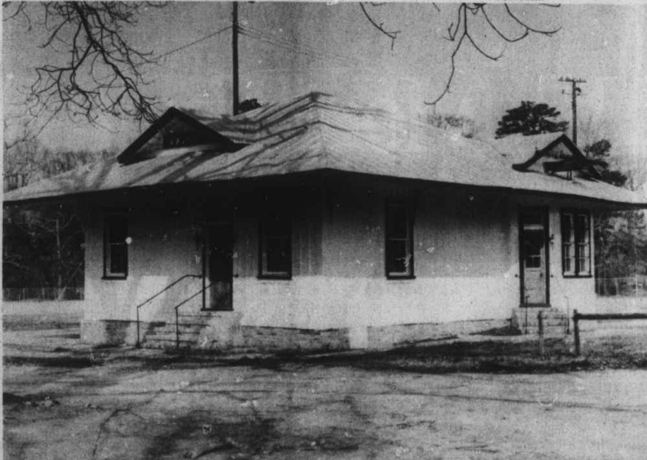
LIBRARY TO OPEN IN HISTORIC DEPOT - The Faison Historical Commission announced tentative plans to open the town library in October. The project to restore the Faison depot began approximately three years ago when the building was donated to the town and moved to the park and recreation grounds. The three-room structure
