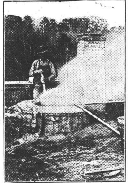
Lime-Sulphur Cooker in Operation.
