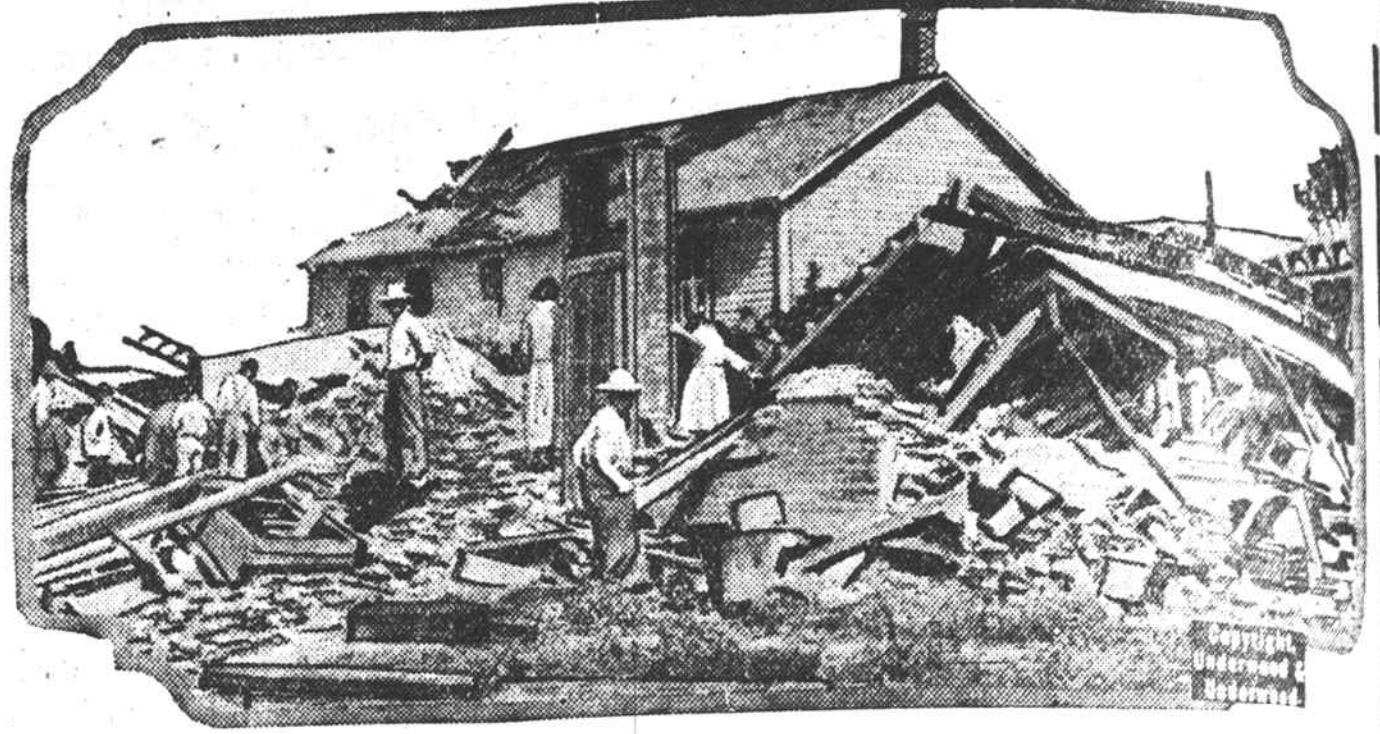
Thirty-five persons were injured seriously by a tornado that swept down on the little town of ... completely demolished many buildings in the business and residential districts. The photograph shows damage on one of the residence streets.
