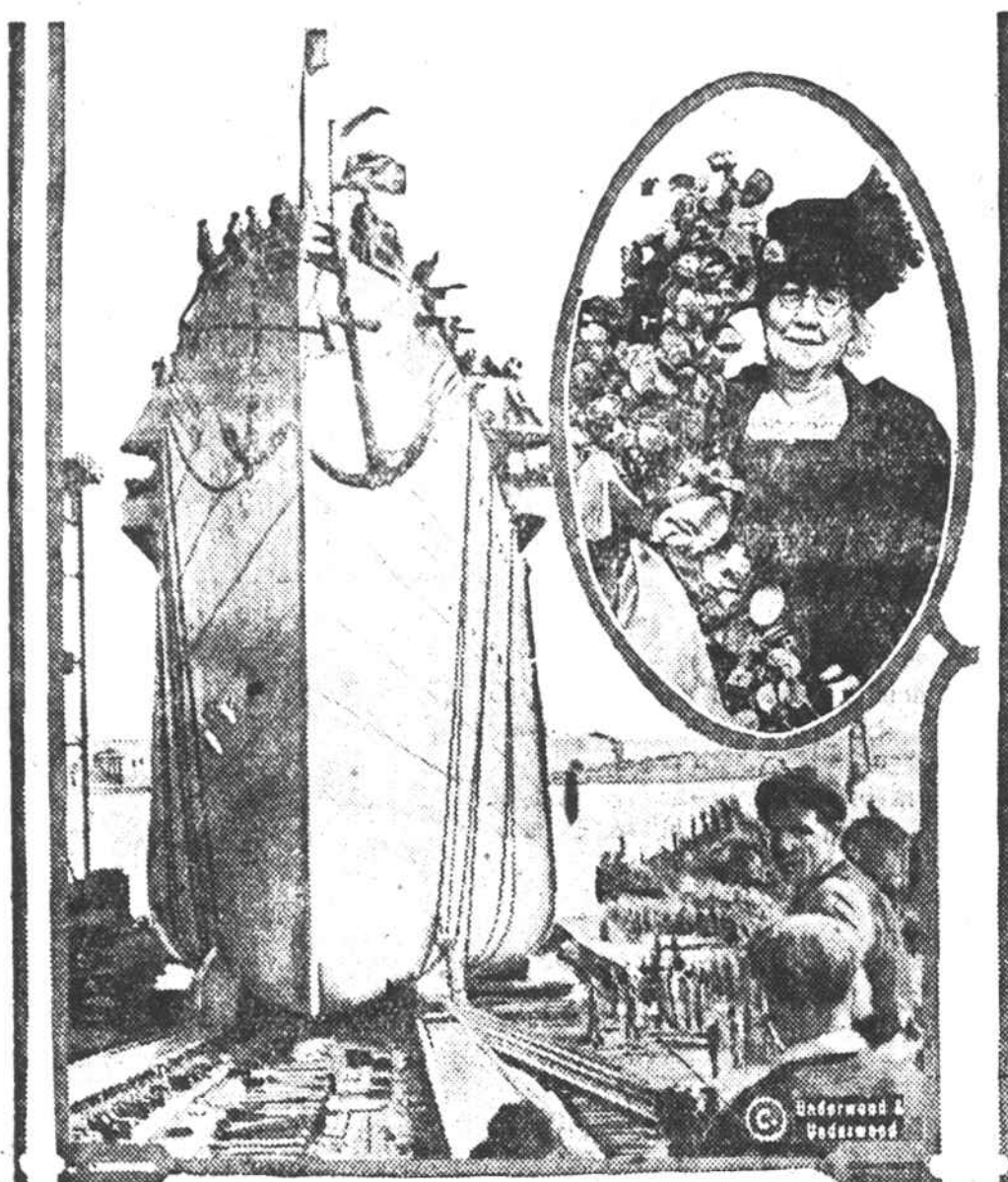
...siding down the ways at the Cramp shipyard, Camden, N. J., is the newest addition to the U. S. navy. Just after she had been christened Marblehead by Mrs. Hannah Martin Evans, mother of the first man from Marblehead, Mass., to meet death in the World war. The new vessel is 555 feet long, 55 feet beam at waterline, and is a combined scout cruiser, flotilla leader, mine layer and airplane carrier. The illustration also shows Mrs. Evans.
