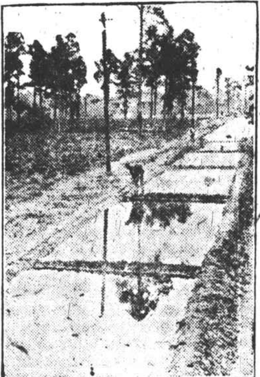
Curing Newly-Laid Concrete by Flooding.
