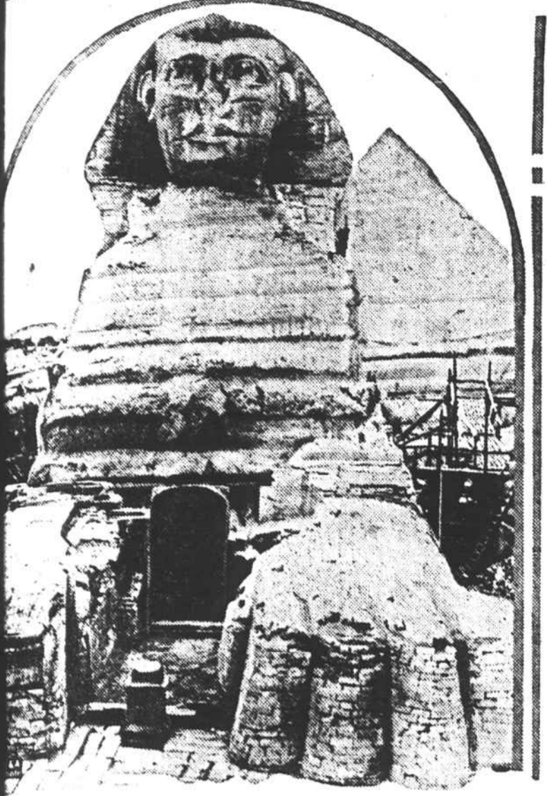
What is believed to be the fourth time in history, the sand has been cleared away from the Sphinx and repairs have been made, even cracks in the head being filled with cement.
