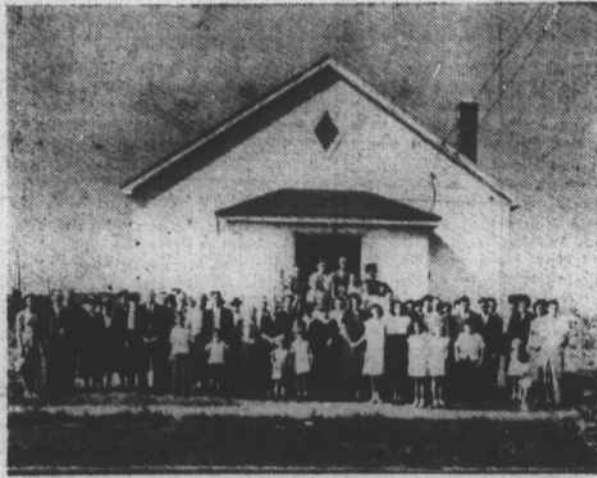
The debt on the newly-constructed First Christian church, Bridges st., Morehead City, was paid in full the last of October. The church was organized last fall by the Rev. C. W. Foster, pastor of the Broad Street Christian church, New Bern.
