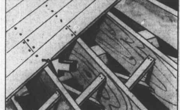
Diagonally laid subflooring adds rigidity. Nails driven on slant pull boards snugly together. Bridging (cross pieces) between joists tends to prevent springy floors.
