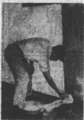
Smooth surface is obtained by second coat in broad strokes with a whitewash or calcimine brush.
