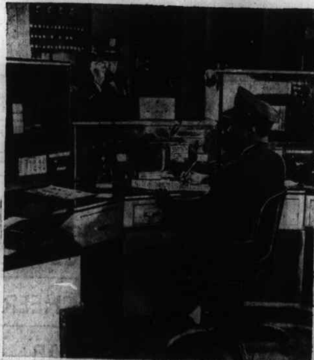
Control room of Pentagon's police department. When guard checks his post, this electronic equipment records it. When something goes amiss automatic warning device alerts operator.
