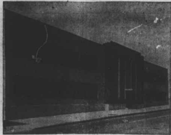
This building is the headquarters, in Charlotte, of the Belk empire. Here, one of every item sold in the Belk stores is on display. Local managers make their merchandise choices, but then buy direct from the manufacturers. Each Belk store is an autonomous unit.
