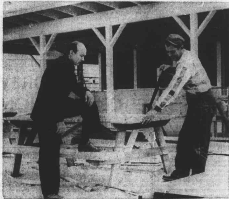
A. B. Cooper, left, and contractor Ty Frost inspect one of the picnic tables that will be in the new park at Moonlight Bay. In the background is a combination shower house-refreshment stand.
