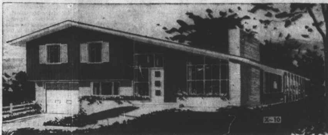
This minimum-sized house has a big house look. Large, four-foot composition panels with square, vertical grooves are used for siding. They go up fast, cutting construction time. Brick is used on the
