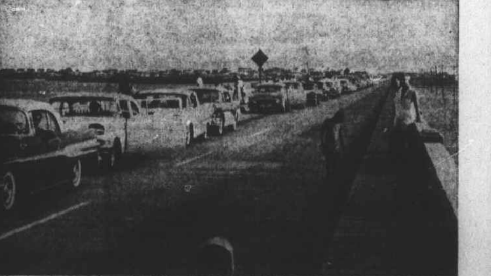
At about 4:30 Sunday afternoon, Aug. 3, a sailboat blew for the Atlantic Beach bridge to open. Because the bridge is the slow-opening, swing type, the bridgetender could not safely close it for part of the auto traffic to pass over, and still re-open it in time to allow passage of a small tug towing two barges. The bridge is so low (13 feet vertical clearance) that even a little tug requires its opening, and automobile traffic was held up for 25 minutes just at the time when homeward-bound weekenders leave the beach. As far as the eye or the camera could see, traffic was backed up. Bridge planners, unfortunately, had not had the foresight to build a higher bridge of the faster-operating bascule type. Photo by Bob Simpson
