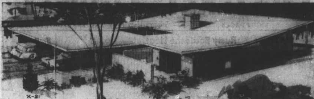
This is an overhead view of the "Roman atrium" house. The private terrace in the foreground is off the master bedroom. The opening in the roof marks the location of the atrium, which is an open interior court exposed to the sky. The front-to-back arrangement makes this an ideal house for a narrow lot.
