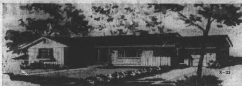
Vertical wood siding is used on all outside walls except for the foyer and living room walls which are finished in brick veneer. White asphalt shingles are recommended for the roof. The garage is at the right, the bedroom wing at the left.
