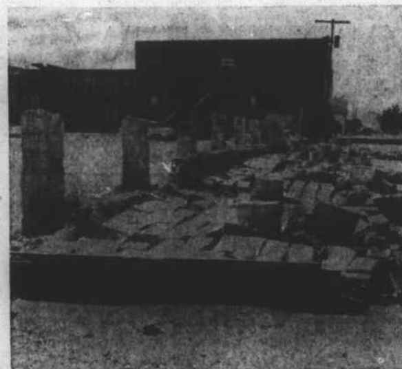
This cement block wall at the west end of the Morehead City High School athletic field was flattened Saturday night.
