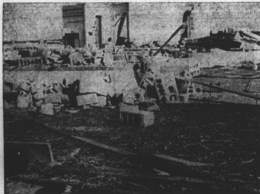
The Dainty Maid Bread Co. warehouse on the Atlantic Beach Causeway was leveled by the force of Helene's high winds. The large front doors blew open and the wind went through the cement block building, taking nearly everything with it.
