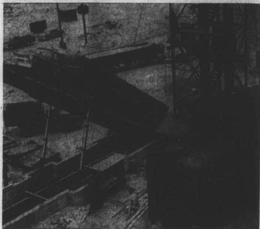
Much of the grain is also brought to the port by truck. Trucks drive onto this device, are weighed and hoisted into this position so the grain will pour off the bed of the truck and into the pit at the bottom of the grain loading elevator.
