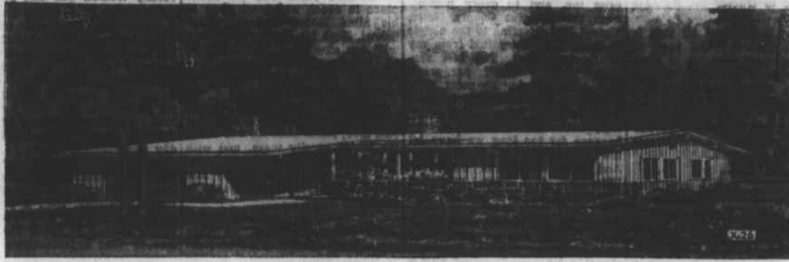
Long and low roof lines, with large overhangs all around, add to the exterior design of this modern adaptation of an original western ranch house. Living and sleeping areas of the house are fully separated.
