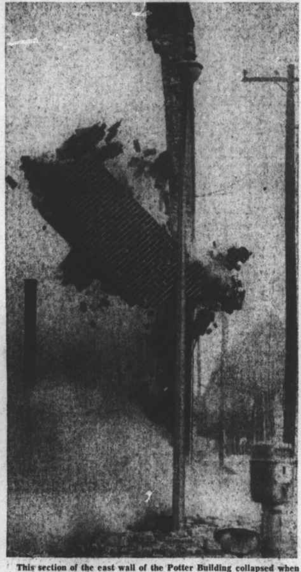
This section of the east wall of the Potter Building collapsed when a Carolina Power and Light truck began to reel in a cable attached to the wall.
