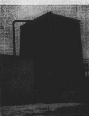
This is the acrator through which all Beaufort water is sprayed. Water is piped from the well in the pumphouse to the top of the aera-tic and is sprayed down into the open tank underseath. Plans call for the tank to be partially enclosed later. Acration removes the hydro-
