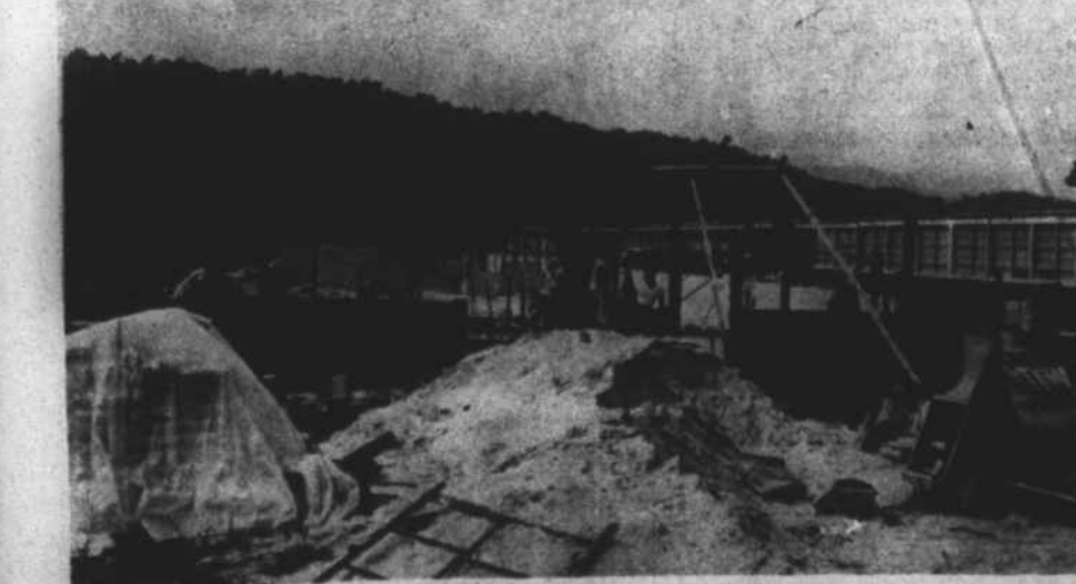
HIGH SCHOOL TODAY - The scene has changed at the Murphy High School in the last month. The walls to the new lunchroom-classroom building are going up at a rapid rate. A covered walkway will connect the new building with the main building. According to H. A. Mattox, chairman of the Murphy School Board, "The board is hopeful that the buildings will be complete in time for school opening this fall. However, this will be ahead of schedule, and depends on the weather and working conditions." (Scout Fot)
