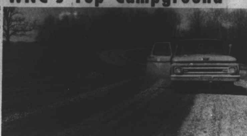
THIS FOREST SERVICE Truck is parked headed out on the driveway which enters the campground area. Concrete 'Ready-Mix' trucks on the hill in the background were pouring the reservoir for the campground's water system on the day this photo was taken.
