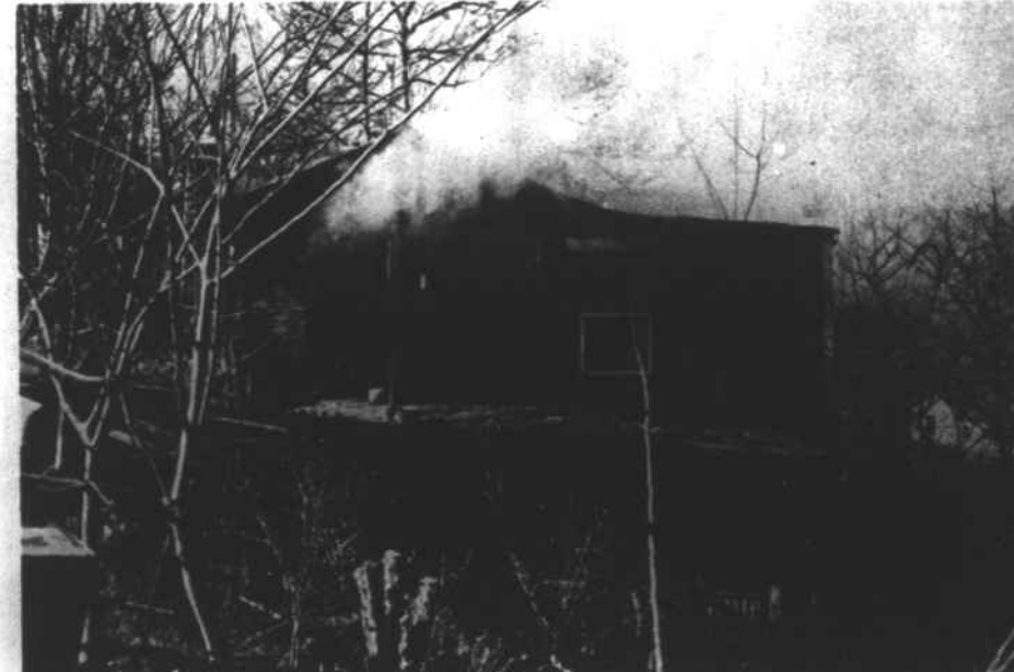
FREEZING WEATHER IS BLAMED for a fire that broke out in the home of Bub Jones on Ridge Street about 12:30 Tuesday, December 1. Mr. Jones said that his water pipes were frozen and that he had been under the house trying to thaw them out with burning newspapers. He didn't discover the fire until after he had gone back upstairs into the house. The fire was confined between a bathroom and bedroom wall. Murphy Volunteer Fire Department extinguished the blaze.
