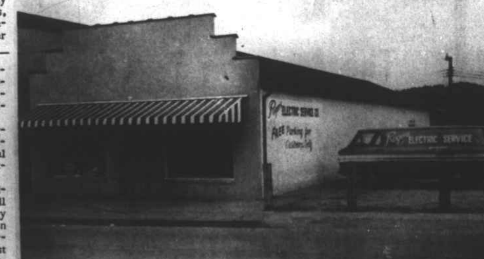
ROGERS ELECTRIC MOVES - Robert Rogers announced this week that they are now in their new location, next door to Hembree's Barber Shop. With almost twice the floor space of their old building, an appliance show room has been added to the new facility.
