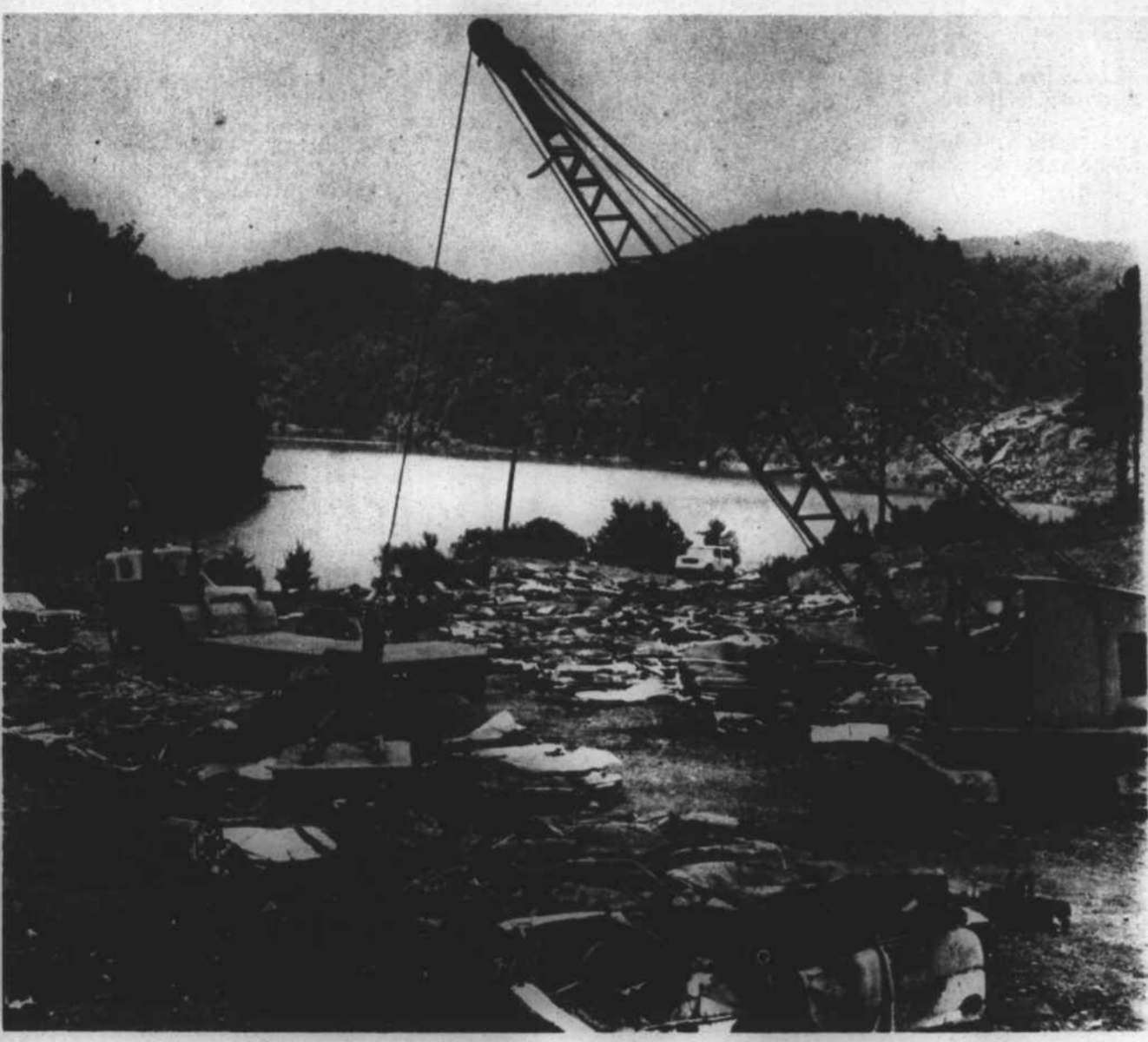
Crane drops 3-ton weight on junk car... flattened bodies then hauled away for scrap.
