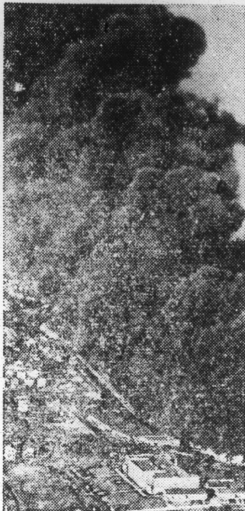
A fire at the Lowenthal Rubber Company in Akron, Ohio, caused a blackout of the city. The firm is in the reclaimed rubber business. Damage was estimated at $50,000.
