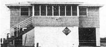
There's a summerplace for you on the oceanfront. Older cottage with 4 BR, 1 bath, 2 half baths, maid quarters on lower level. $89,900.
