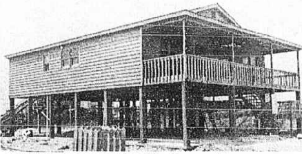
UNDER CONSTRUCTION—Brunswick Ave. Large 4-BR, 2-bath home with C/H/A, dishwasher, front covered porch, large screened porch and open deck. $99,500.
