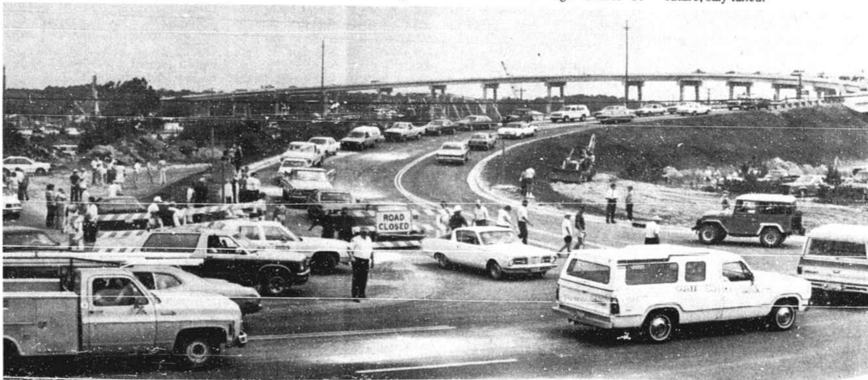
MODERN HIGH-RISE BRIDGES opened at Ocean Isle Beach in 1985 and at Holden Beach (pictured) in 1986.
