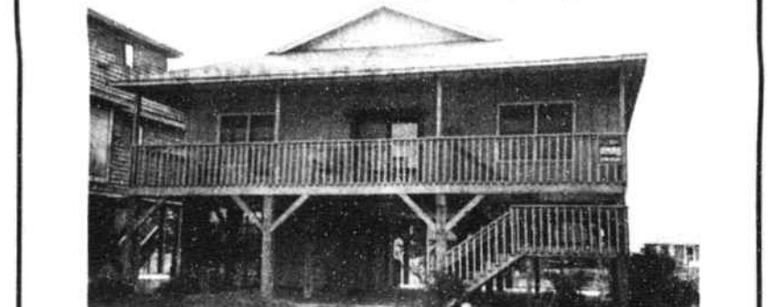
256 EAST SECOND ST. -Third row cottage with 3 BR, 3 baths. Large deck, completely furnished, easy beach access. $119,900.
