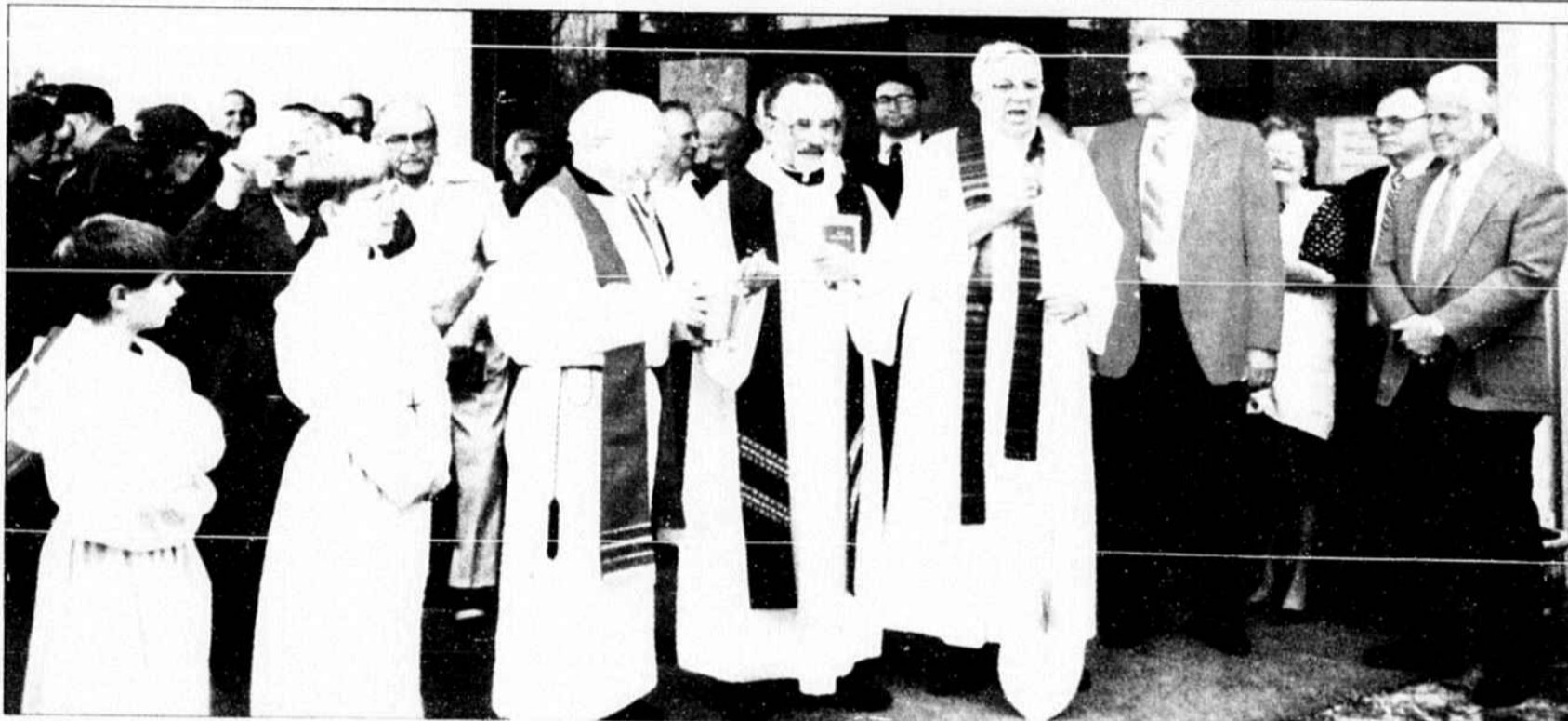
Breaking Ground At St. Brendan's
