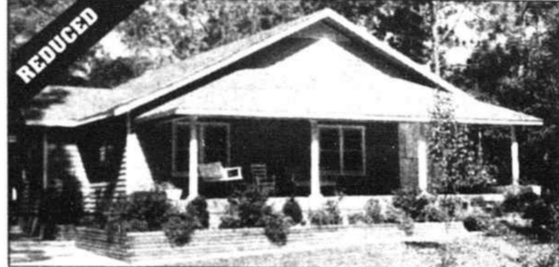
CLASSIC CHARM, 1008 HIGH POINT AVE. —Front porch stretches across front of home, back porch is screened and private. Open floor plan with over 1700 sq. ft. and lots of tile, skylights, BR, fireplace, hardwood floors and new carpet. 3 BR, 2 baths, extra sitting room, many extras including large wood corner lot. Convenient location. REDUCED $129,900.
