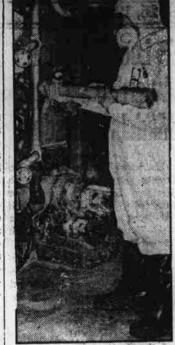
ATOM AGE PLUMBER— Technician at the Hanford Atomic Products Operation, Richland, Wash., carries a meter instead of a monkey wrench when searching for leaks in "hot" plumbing. The GE-de-veloped device employs a sodium iodide crystal, light output of which under atomic radiation is measured on a light-type meter at end of barrel.
