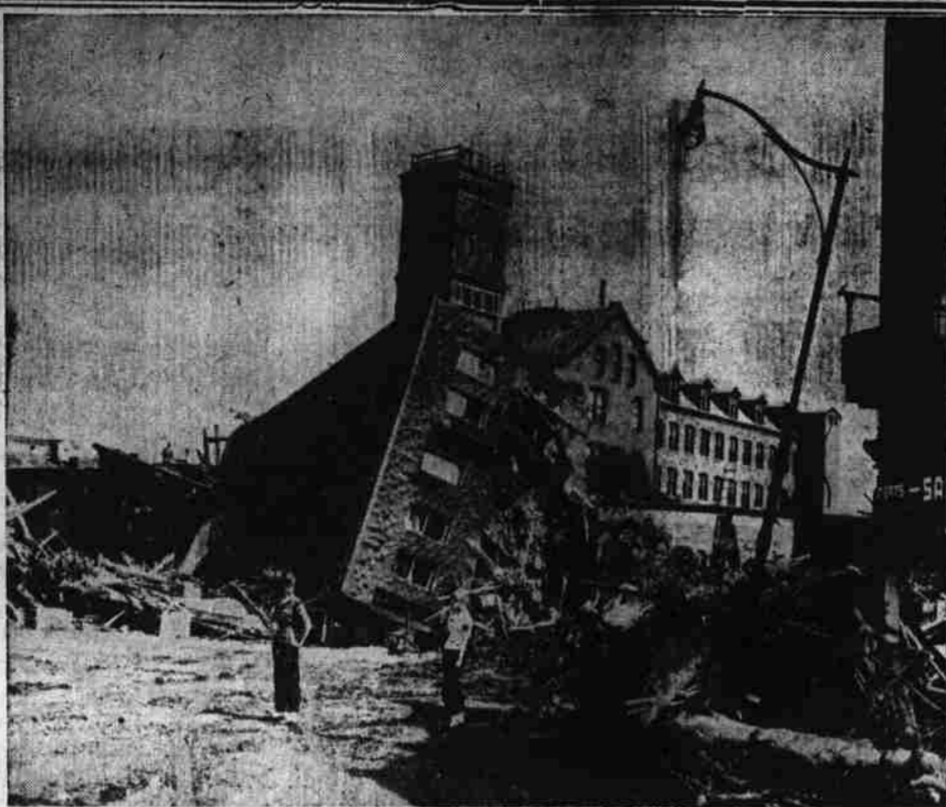
CRUSHED AND BROKEN, this 16-family apartment house in Waterbury, Conn., was left high in the flood which, according to the Red Cross, destroyed 1,326 houses and badly damaged 4,808. (Wide World Photo)
