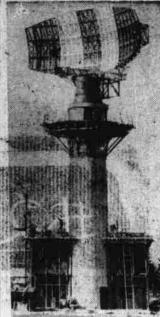
SKY SENTRY - Set to start scanning the skies in the near future, a giant radar tower nears completion in Munich, Germany. The tower features a six times a minute from its 70foot-high perch It is capable of "viewing" all air traffic for a radius of 330 miles and up to 13 miles altitude.
