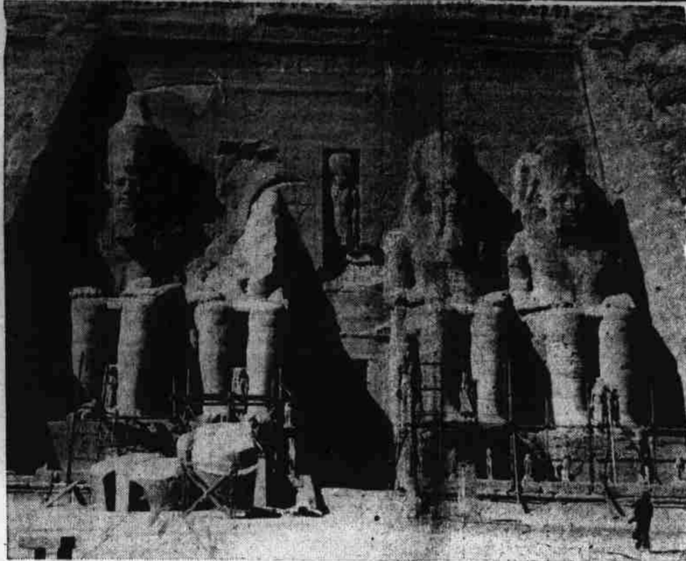
WILL THEY SAVE IT?—Archeologists and engineers are wondering how this ancient temple in Luxor, Egypt, can be saved. The structure, built by Rameses II, 3,000 years ago, rests on sand destined to be covered by waters backed up from the nation's Aswan dam. Suggestions range from creating a special dam around the temple to moving it elsewhere stone by stone.
