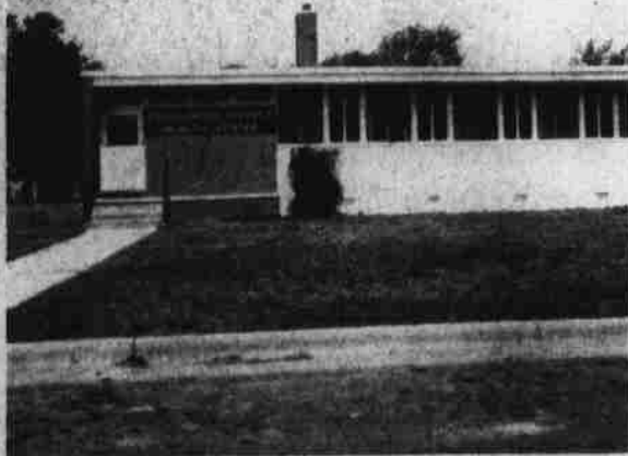
NEW STATUTES —The '73 General Assembly has enacted several laws designed to boost the ability of the local health departments across the state to boost their services. According to district health director, Howard Campbell, this district is following through on the new laws.
