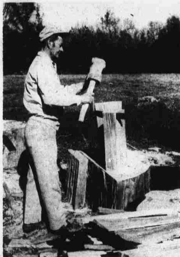
DEMONSTRATION — W.D. Kemp, restoration constructor for the Newbold-White House demonstrates the way the shingles are being made with the same tools early settlers used, a frow and a mallet.
