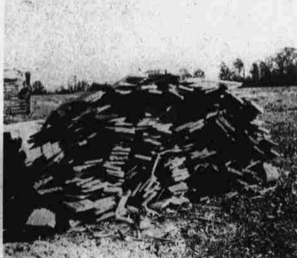
FINISHED — Shown here is a pile of the finished shingles which will be used on the roof of the Newbold-White House. Shingles for this purpose have not been hand-split in Perquimans County in at least 100 years. (Staff Photos by Kathy Newbern)
