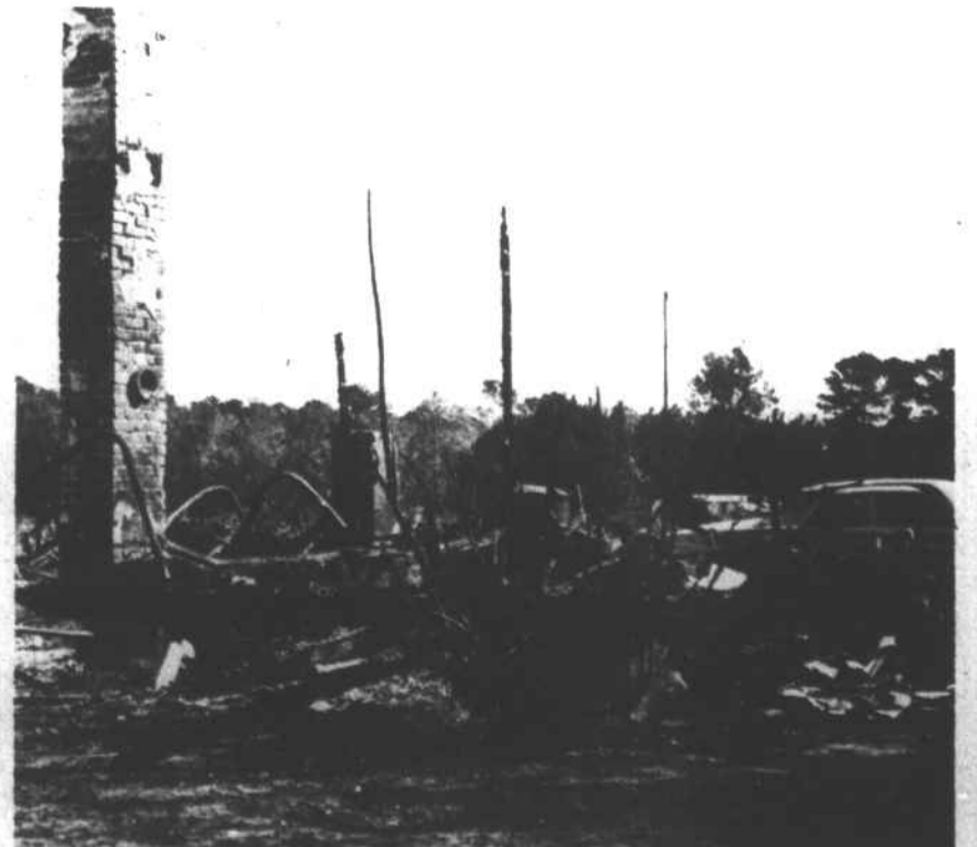
LOCAL FIRE — A fire broke out early Saturday morning completely destroying a house across from Wynne Fork Courts outside of
