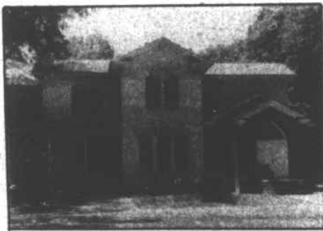
Swindell Funeral Home-Original Building
