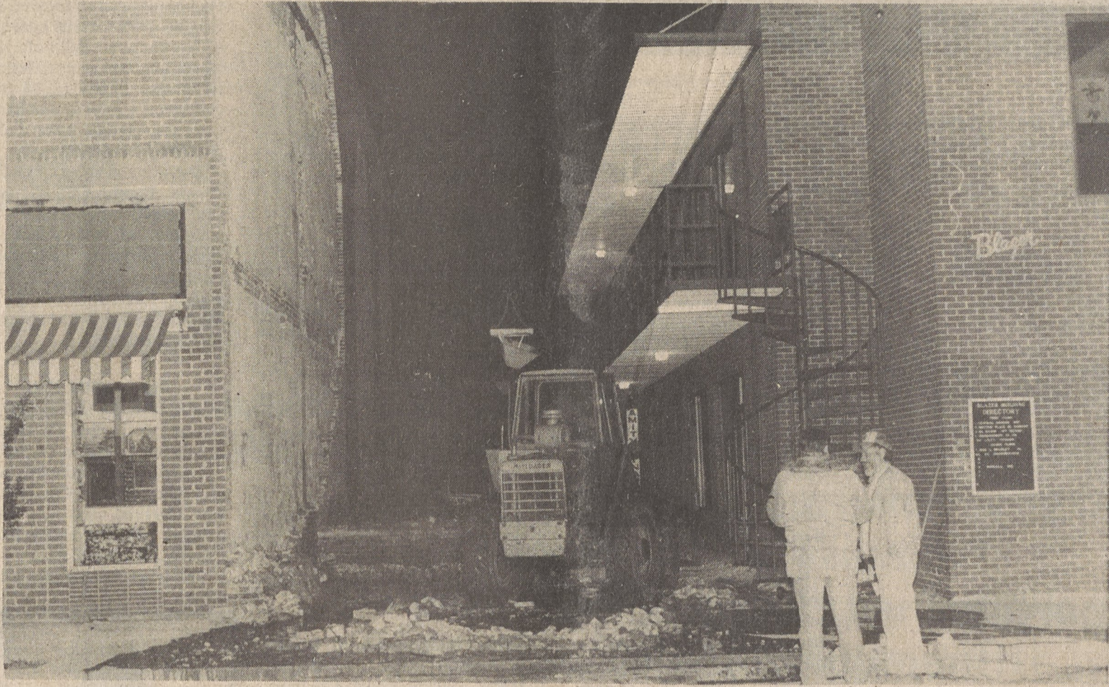
City crew cleans up destroyed wall....
